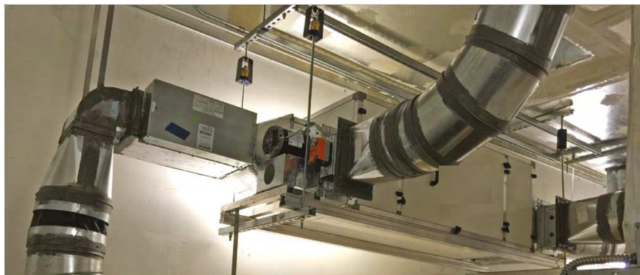
Figure 3: Energy WELL module installed at the University of Miami.
